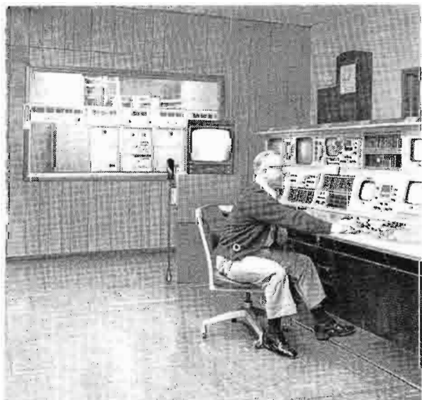
Through the picture window, production control operator has a clear view of transmitter control/metering panels.
